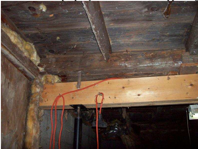
This is another view of the shoring beam.
